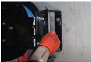
Insert the swivel rod through the holes of the base plate and swivel arm plate.
