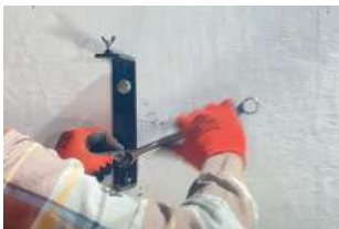
Secure the mounting plate with load-rated fasteners suitable for the wall and environment.
