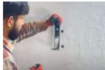
Mark two holes on the wall for the base plate.
