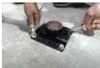
Insert lag shields in holes and place bottom plate over the holes.
