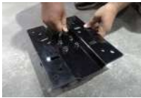
Use lag screws to attach bottom plate to the floor.
