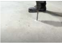
Drill holes in floor.
