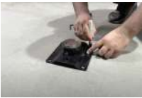
Place bottom plate on floor and mark holes.
